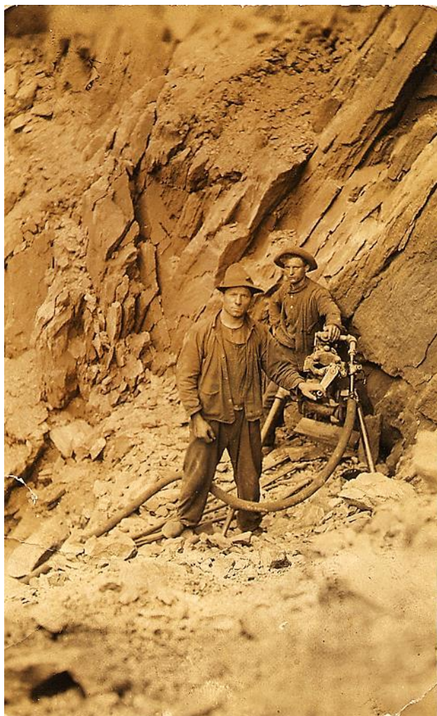
East Chapin Miners with a Rand Drill, 1916
