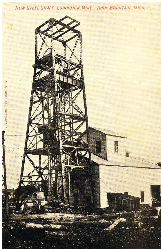
New Steel Shaft, Ludington Mine, Iron Mountain, Mich., showing building housing the Cornish Pumping Engine ca. 1908-1910
