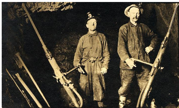
Postcard of two miners with Rand Drills, possibly in the Millie Mine, ca. 1907-1920
