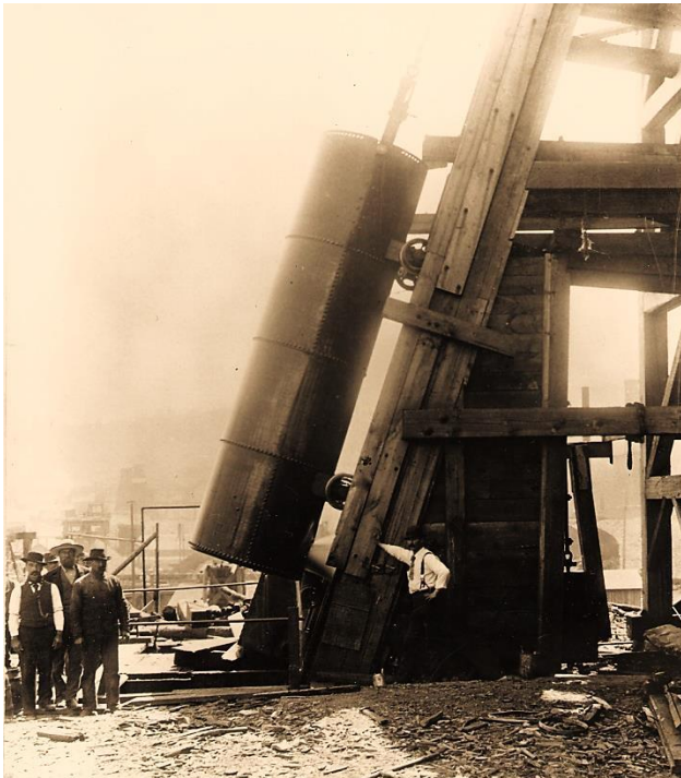
This photograph shows the 2,650-gallon bailer used to dewater No. 2 Shaft of the Hamilton Mine
